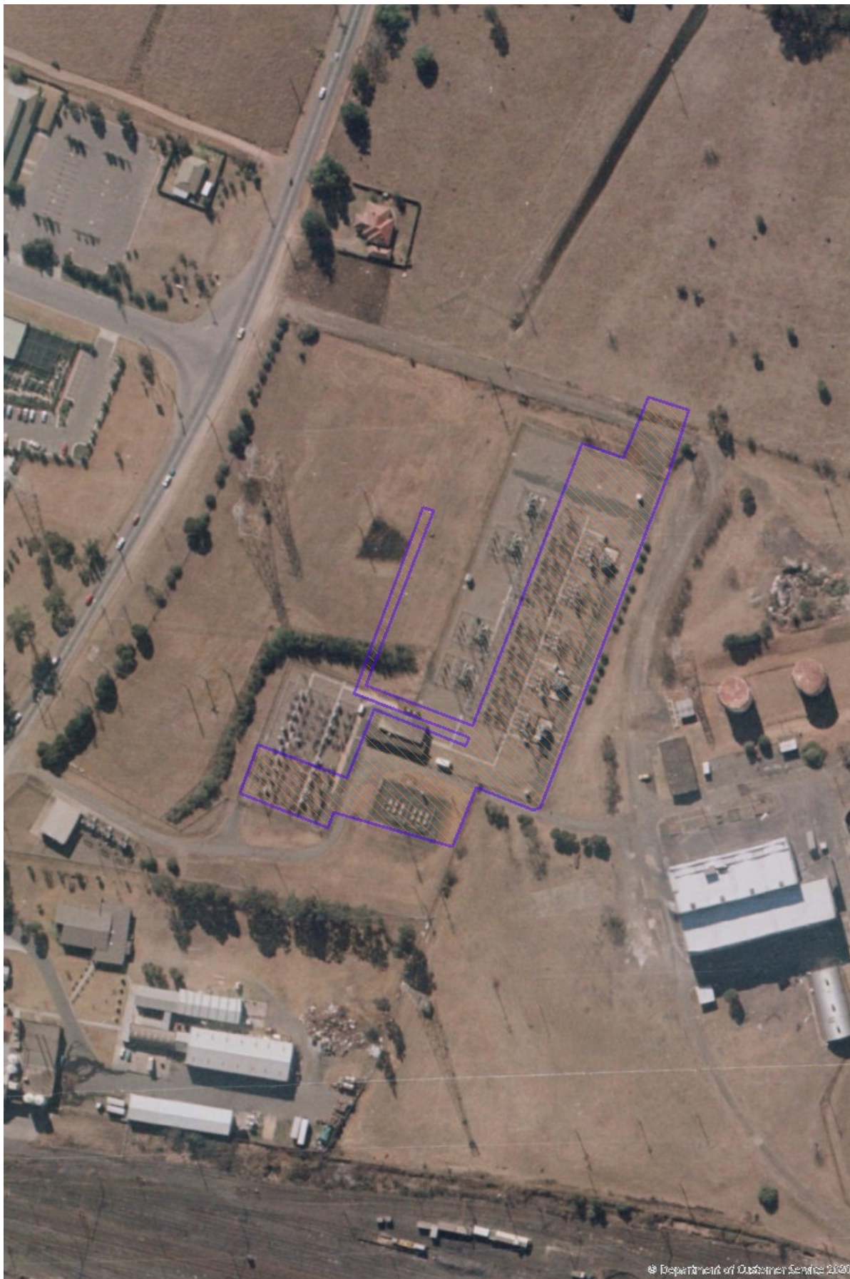
Figure 4-3 1986 Land used as Substation and Switchyard
