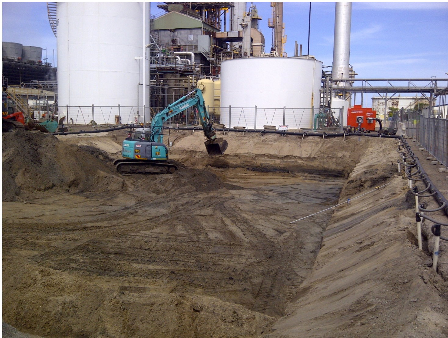
Figure 8 Excavation with installed dewatering system
