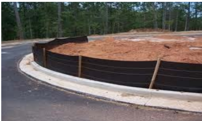
Figure 12 Sediment and erosion control in place
