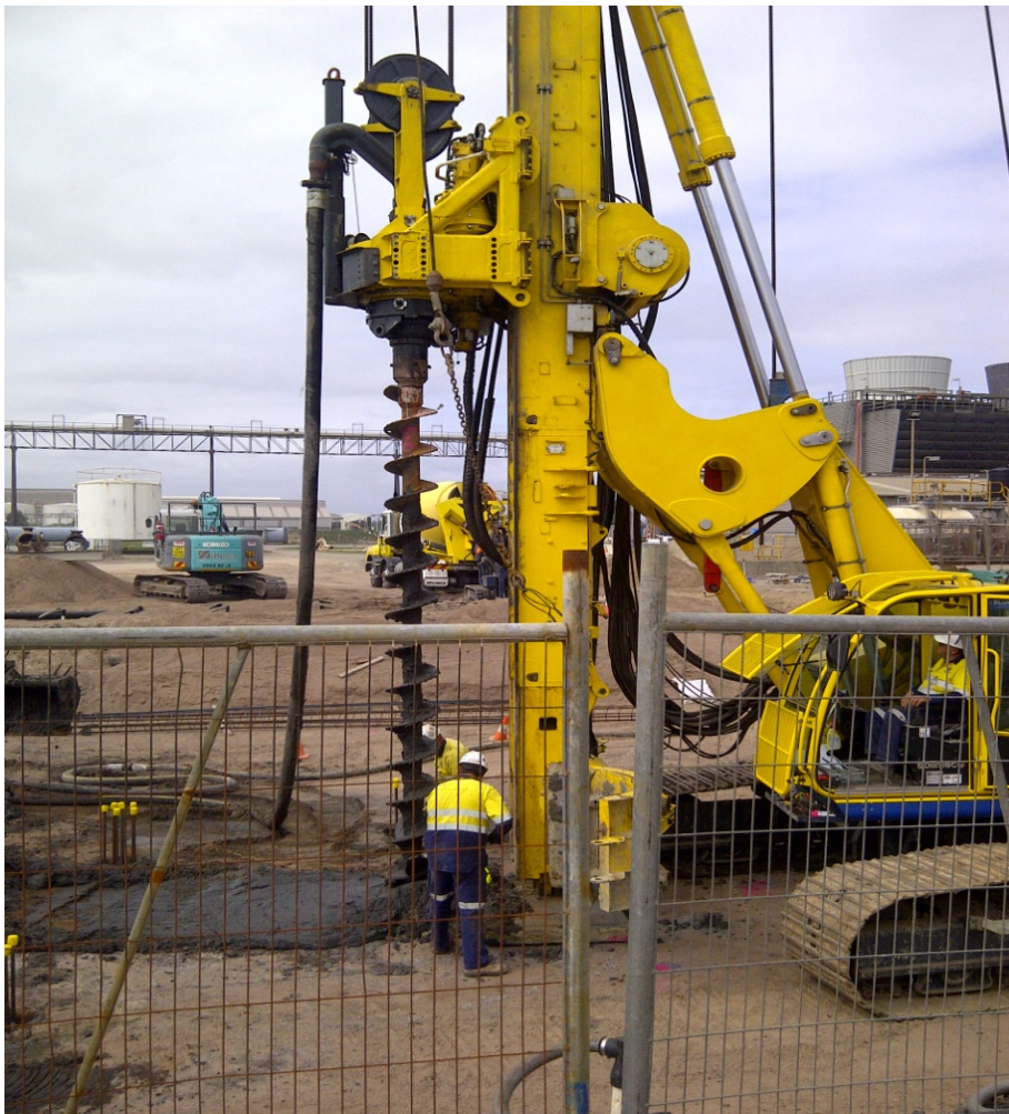
Figure 10 Noise generating equipment
