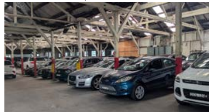
INTERNAL TIMBER STRUCTURE
