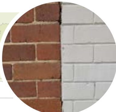
EXISTING SITE BRICKS
