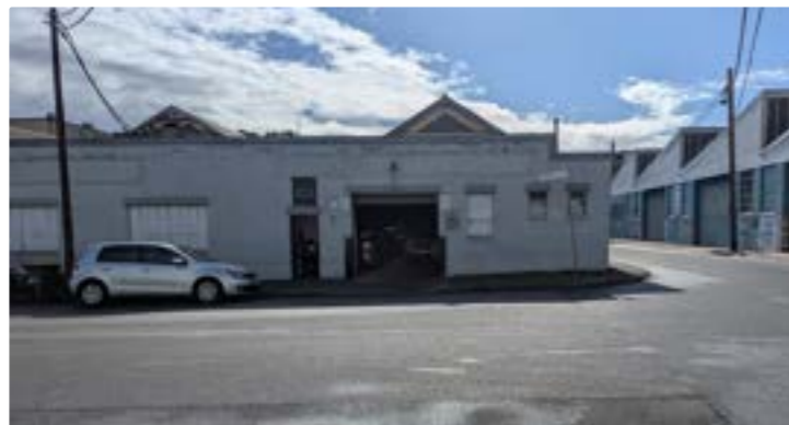
SOUTH SITE & WILLIAM ST VIEW WAREHOUSE ROOFLINE
