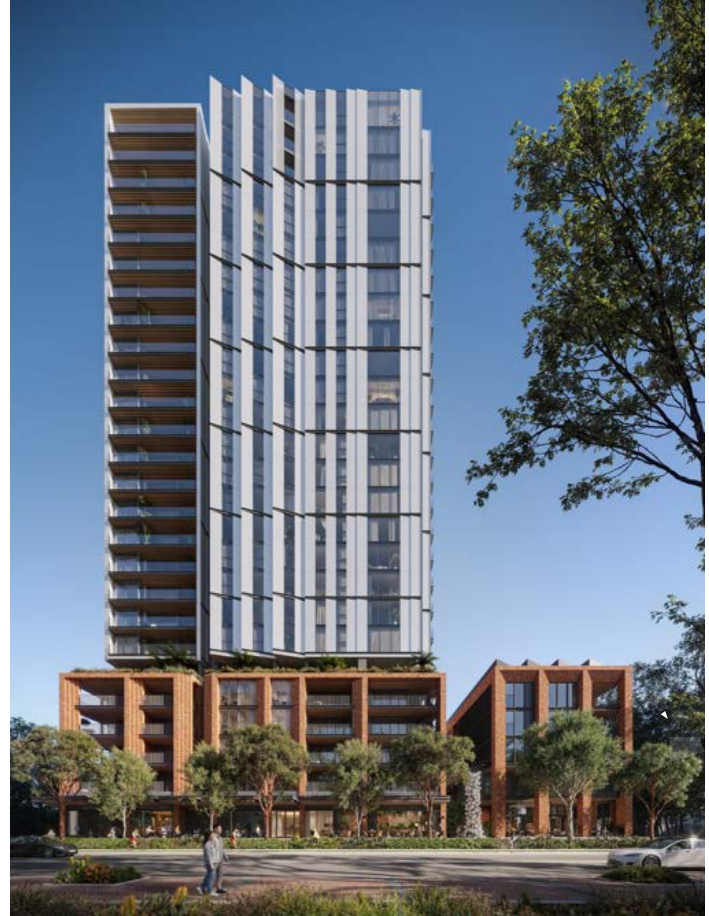
EAST ELEVATION - VIEW TO WEST
