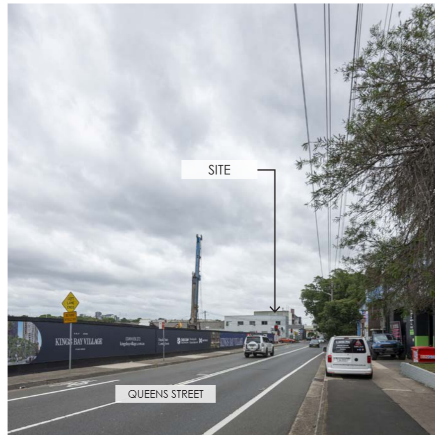
View looking west from Queens Street
