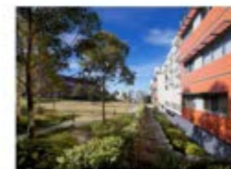
Figure 4O.4 Shading trees improve the microclimate and are particularly effective along the eastern and western elevations of buildings.
