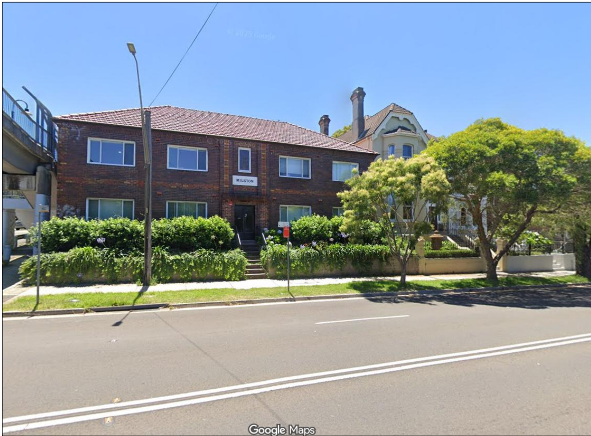
Figure 51: Existing elevated residential properties along northern end of Stanmore Road (Source: Google Street View)
