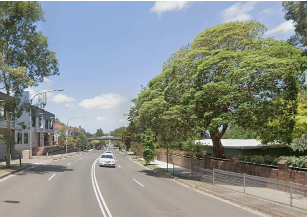
Existing footbridge over Stanmore Road retained
