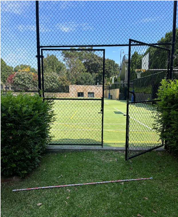
Figure 23 – North-West view of Sevington Courts entrance.
