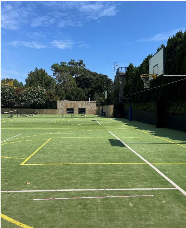
Figure 25 – West view of Sevington Courts. Note presence of retaining walls along the Northern and Western bounds of the site.
