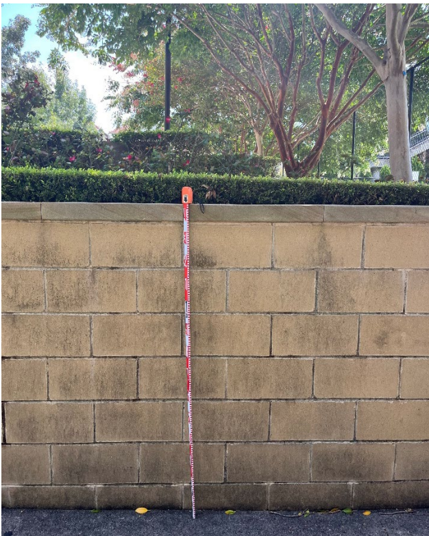
Figure 29 – North view of retaining wall for the terraced garden to the west and south-west of Sevington Courts.
