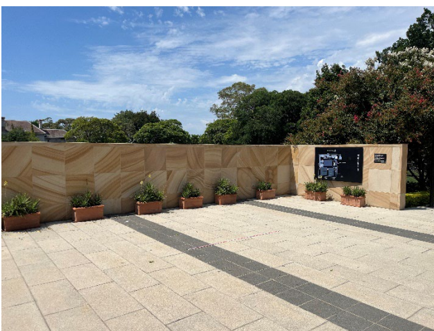
Figure 35 – South-east view of the main (paved) walkway accessible from Stanmore Road (west of Sevington Courts).
