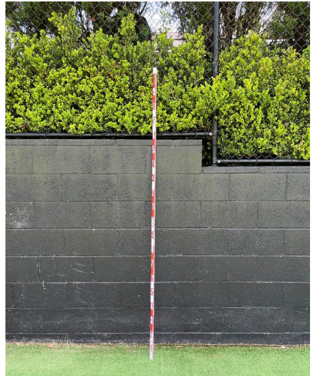
Figure 26 – Retaining wall along the northern boundary of the Sevington Courts.
