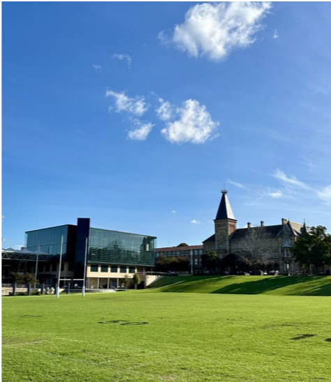
6. Views across Johnson Oval towards Founders Building and Rae Centre
