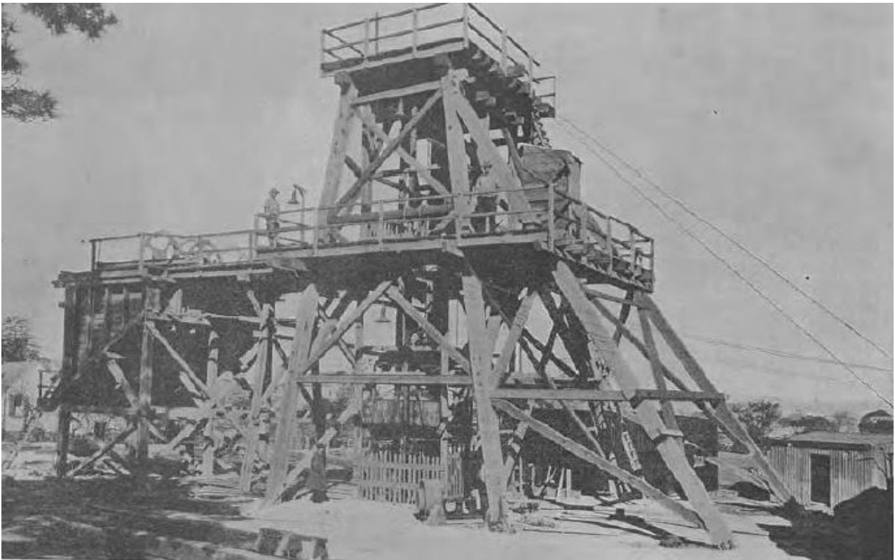
Figure 16 – Historical image of 'Shaft 13' located at the site of the present tennis courts. Construction involved extensive ground disturbing processes.
