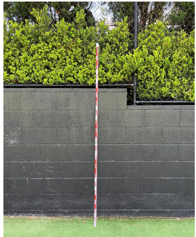
Figure 27 – Retaining wall along the northern boundary of the Sevington Courts.
