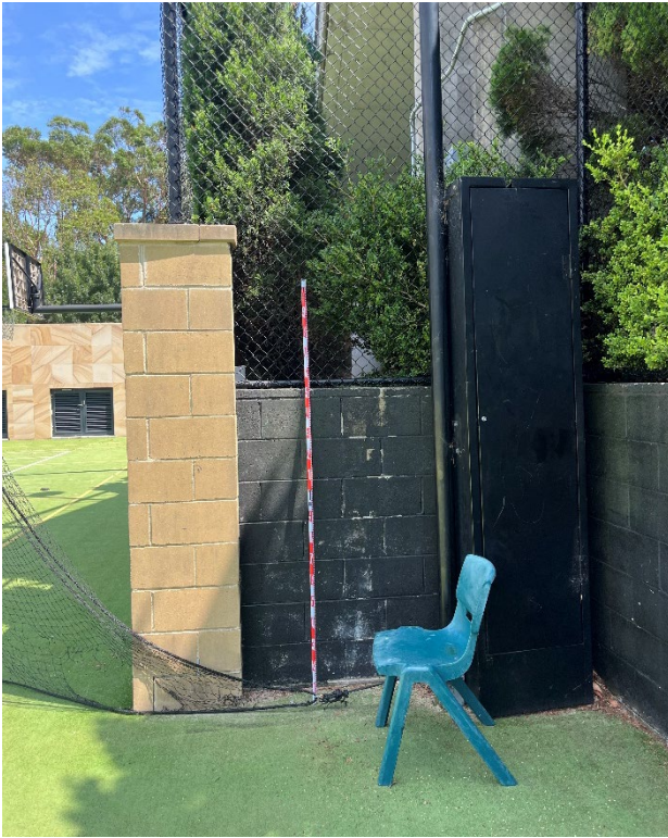
Figure 28 – Retaining wall along the north-western boundary of the Sevington Courts.
