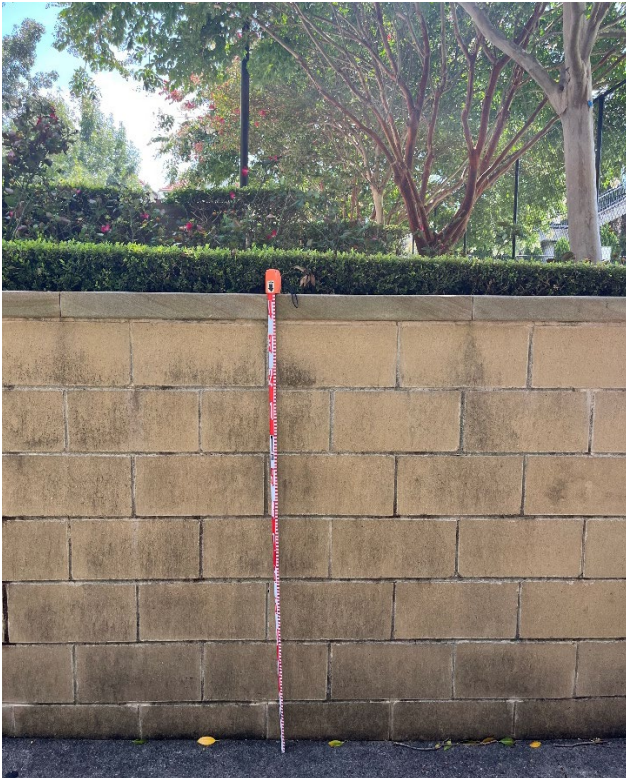
Figure 30 – North view of retaining wall for the terraced garden to the west and south-west of Sevington Courts.
