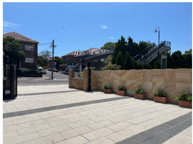
Figure 37 – Northward view of the main (paved) walkway accessible from Stanmore Road (west of Sevington Courts).
