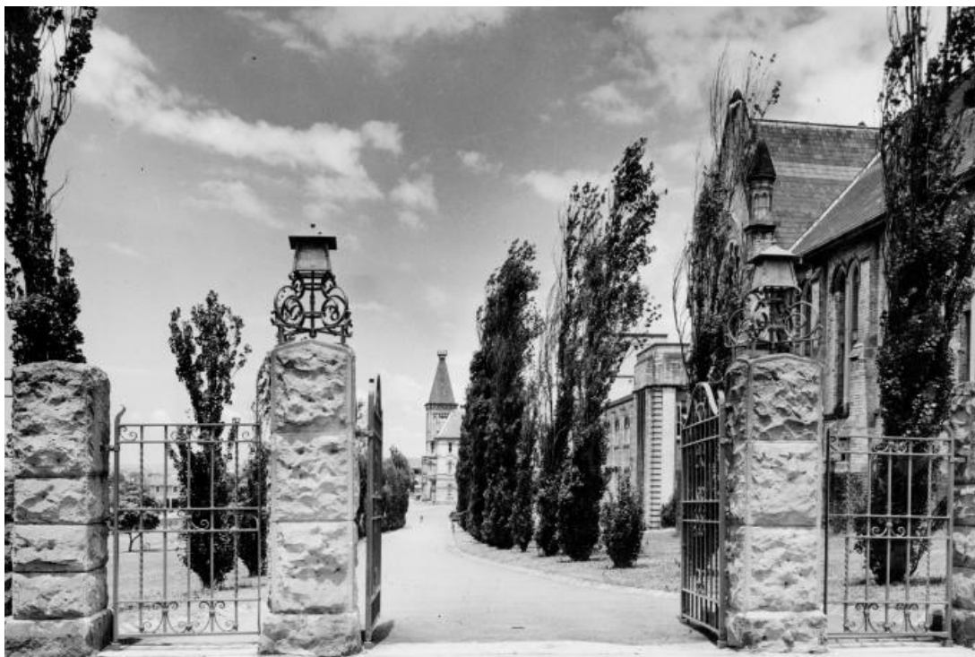
Figure 2.13 – Millner Gates and Memorial Drive circa 1960 (Photo: Newington Archives)
