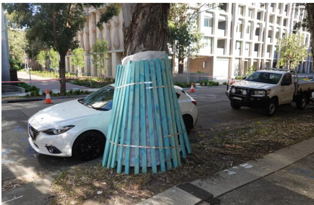
Figure 3.3 – Example of acceptable Trunk Protection batten installation. (Photo: Arterra)
