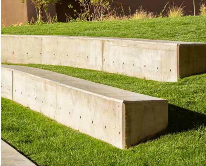
CONCRETE TERRACES EASTERN OVAL BOUNDARIES
