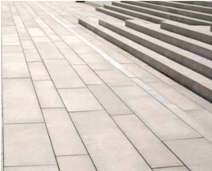
CONCRETE UNIT PAVING MAIN PEDESTRIAN WALKWAYS
