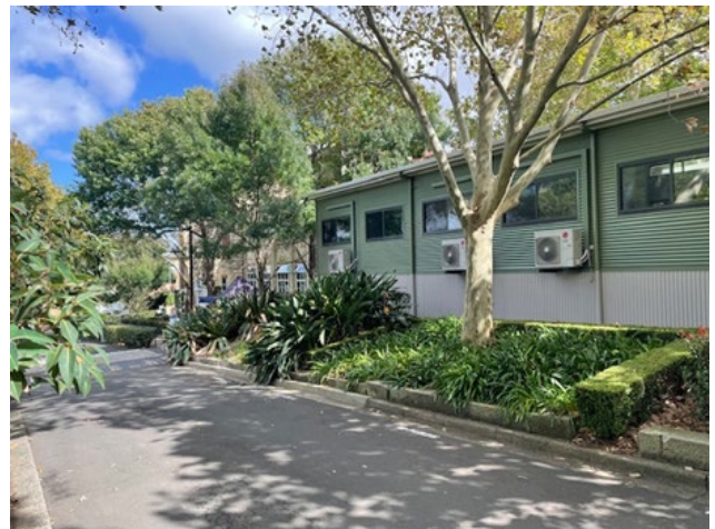
Figure 63 Temporary demountable classrooms.
