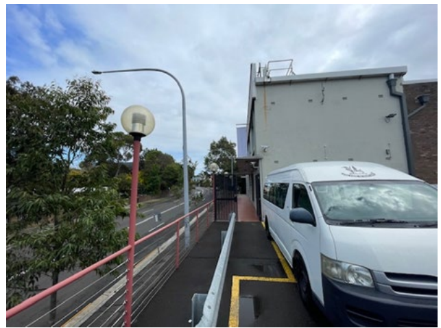
Figure 67 Upper-level car park to the Concordia Building.
