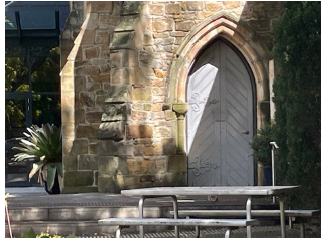
Figure 39 Timber door with stone hood mould.
