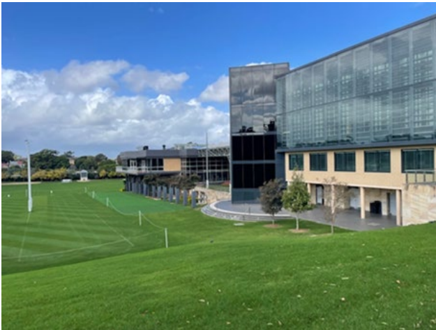
Figure 58 Northern elevation of Rae Centre and Taylor Sports Centre facing Johnson Oval
