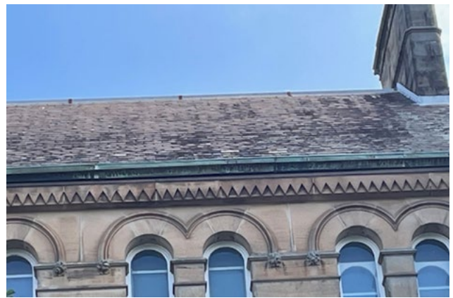
Figure 25 Slate roof viewed from east elevation.
