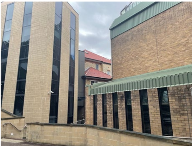
Figure 62 Western elevation of the Tupou Centre which is located adjacent to the chapel.
