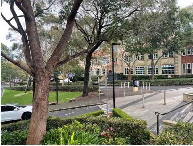
Figure 15 Entrance to the Stanmore campus from Stanmore Road.
