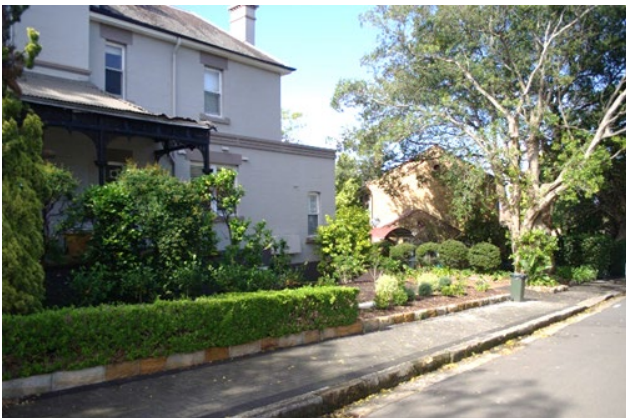
Figure 42 South-western elevation of the Parsonage showing landscaping and driveway to the rear of the site.
