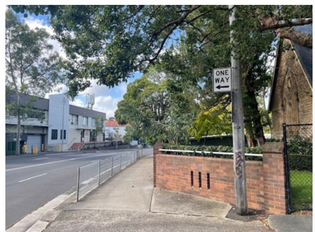
Figure 37 Surrounding context, showing later wall separating site to Stanmore Road.
