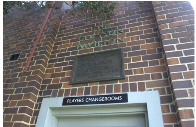
Figure 55 Brick exterior wall of amenity block entrance, showing signage.
