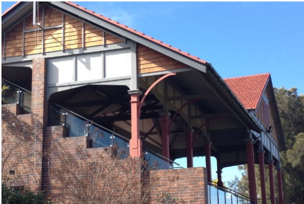
Figure 54 Timber and tiled roof of Glassons Pavilion
