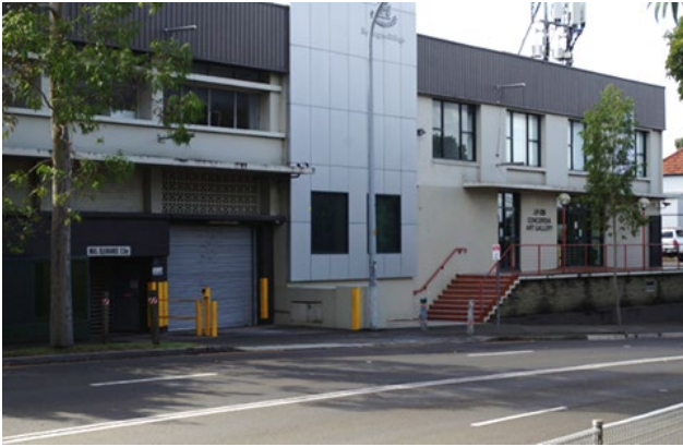
Figure 64 Southern elevation of Concordia Building facing Stanmore Road
