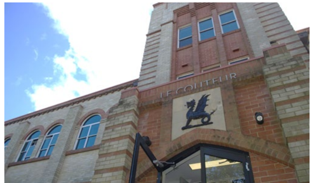
Figure 47 Central entry tower showing the brick detailing.
