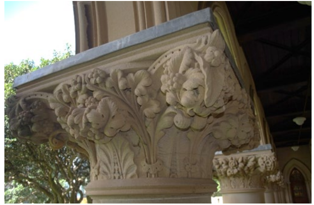
Figure 23 Stone detailing of loggia column capital.
