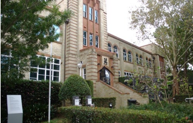
Figure 44 Eastern elevation of the Le Couteur Centre as seen from the southwest
