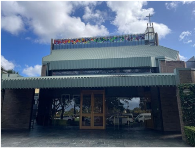
Figure 52 Main entrance of the Chapel, seen from the south-east.
