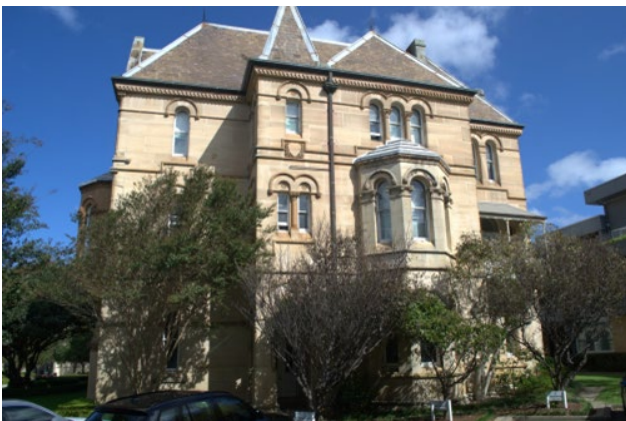
Figure 18 Northern façade of building, showing bay window and conjoined towers.
