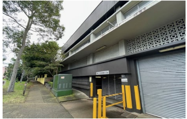
Figure 65 View from street looking to the west to Concordia Building on Stanmore Road
