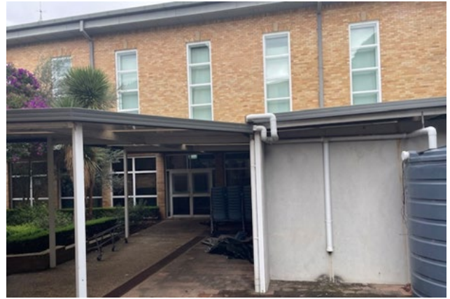
Figure 49 Western elevation (rear entrance to the Centenary Hall)
