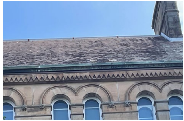
Figure 26 Slate roof viewed from east elevation.
