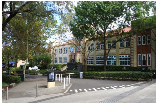
Figure 14 Le Couteur Centre Building and formal pedestrian walkway as accessed from Stanmore Road.
