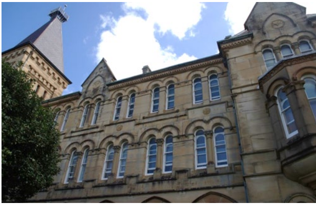
Figure 21 Main eastern façade of building, showing arched windows and decorative stone banding.
