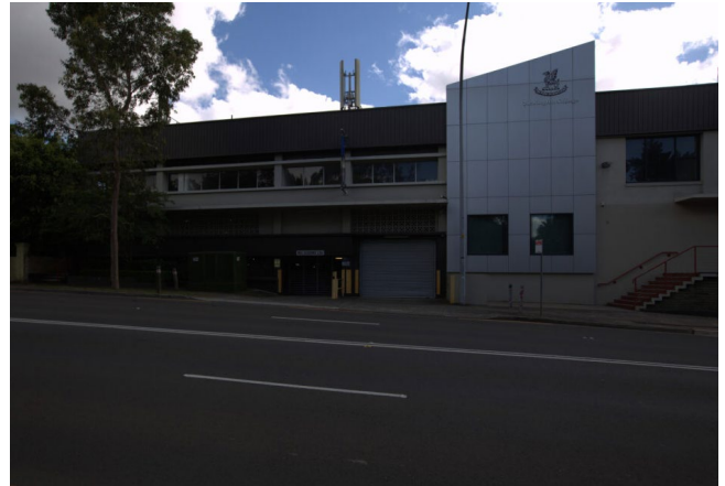
Figure 84 View of the front façade of the Concordia Building, to Stanmore Road.
