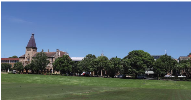
Figure 88 Existing view towards Centenary Hall.
