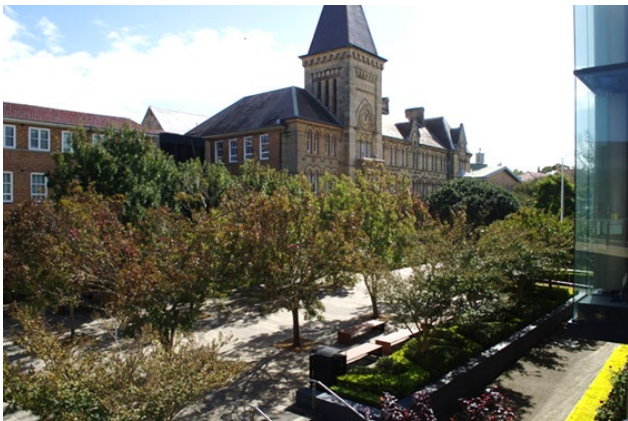
Figure 13 Formal pedestrian walkway and Founders Wing.
