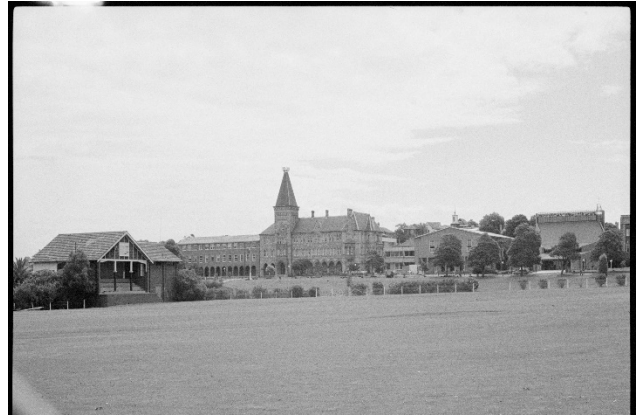
Figure 69 View from Johnson Oval, looking west, 1987.
