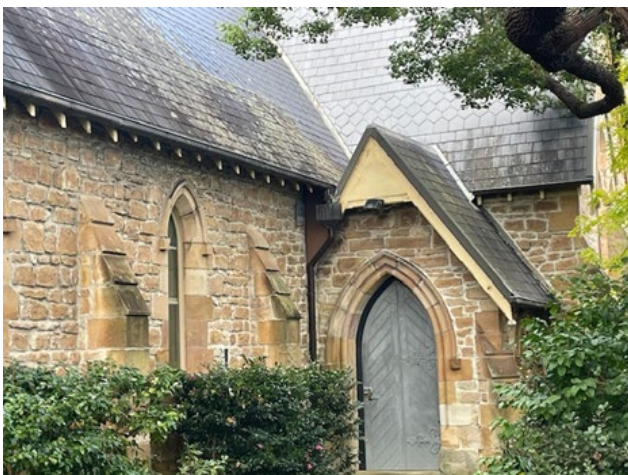
Figure 39 View of the transept entrances on the western façade.
