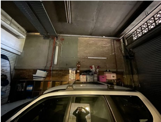
Figure 53 Garage in Concordia Building.
