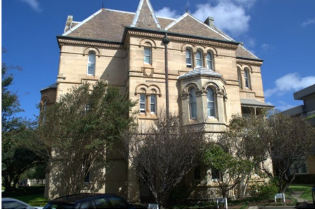
Figure 19 Northern façade of building, showing bay window and conjoined towers.
