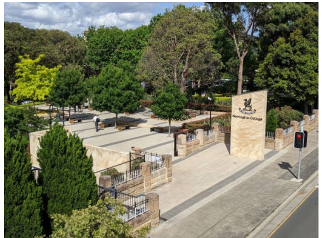
Figure 11 Entry forecourt to Stanmore Road
