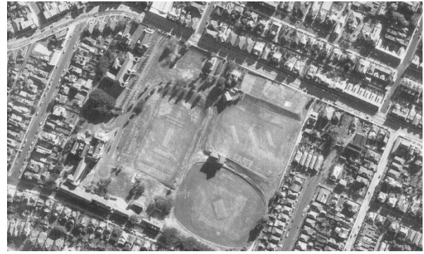
Figure 5 Historical aerial shown Johnson Oval, c.1943.
