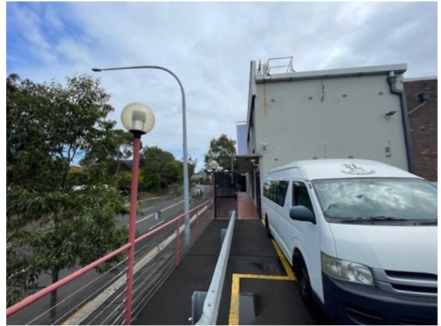
Figure 52 Upper-level car park to the Concordia Building.
