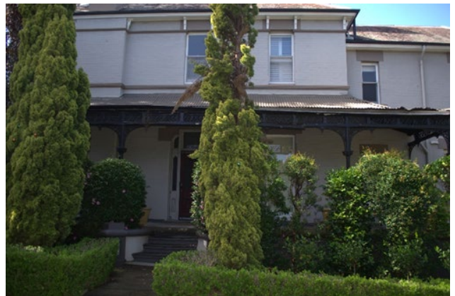
Figure 42 View of western elevation showing the covered entryway and entrance door.
