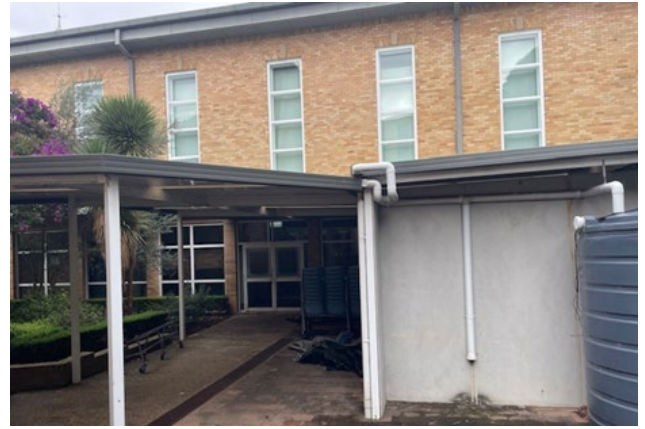
Figure 46 Western elevation (rear entrance to the Centenary Hall)
