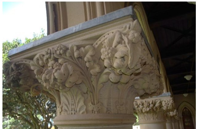
Figure 24 Stone detailing of loggia column capital.
