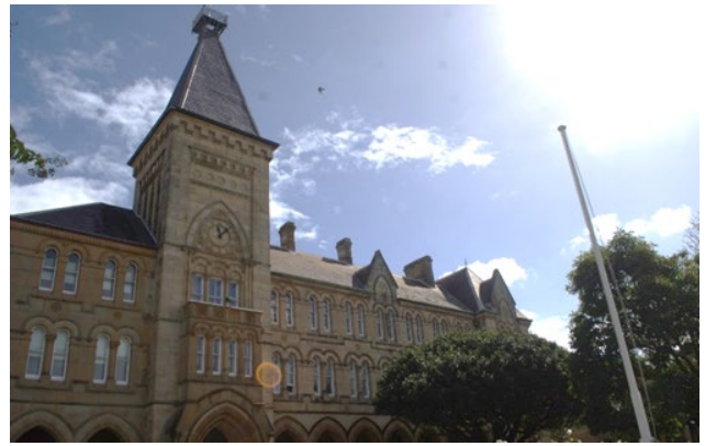
Figure 22 Main eastern façade of building showing clock tower.
