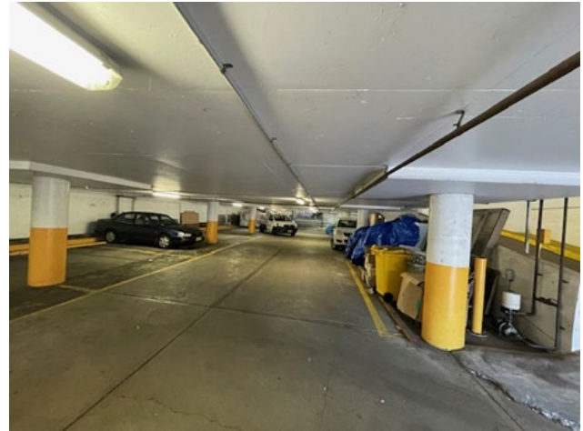
Figure 54 Car park in Concordia Building.
