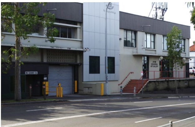
Figure 49 Southern elevation of Concordia Building facing Stanmore Road
