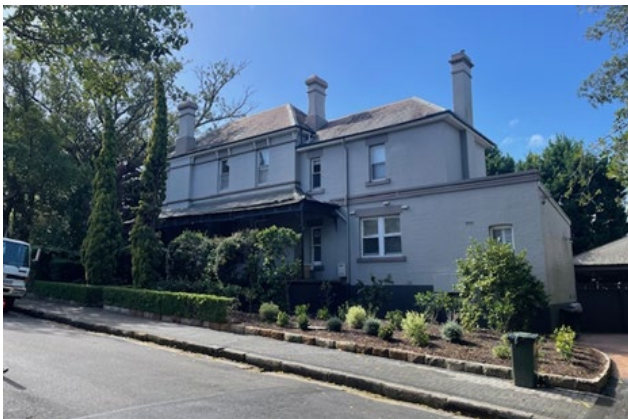
Figure 41 Western elevation as viewed from entrance road off Stanmore Road
