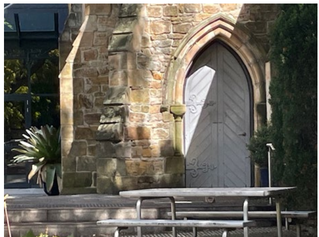
Figure 40 Timber door with stone hood mould.
