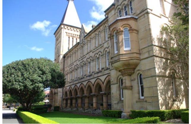
Figure 20 Main eastern façade of building, showing oriel window.
