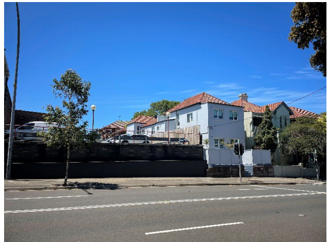
Picture 4 View north-east across Stanmore Rd to location of the future arts facilities
