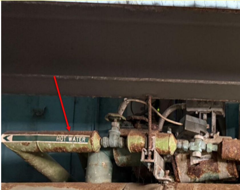
Photo 1: Assumed SMF insulation for HVAC system in Centenary Hall
