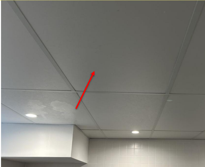
Photo 2: Assumed SMF ceiling tiles in bathrooms, classrooms and offices in Centenary Hall
