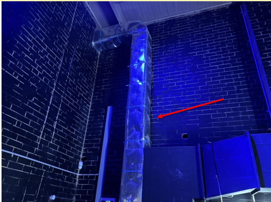
Photo 1: Assumed SMF insulation for HVAC system in Centenary Hall
