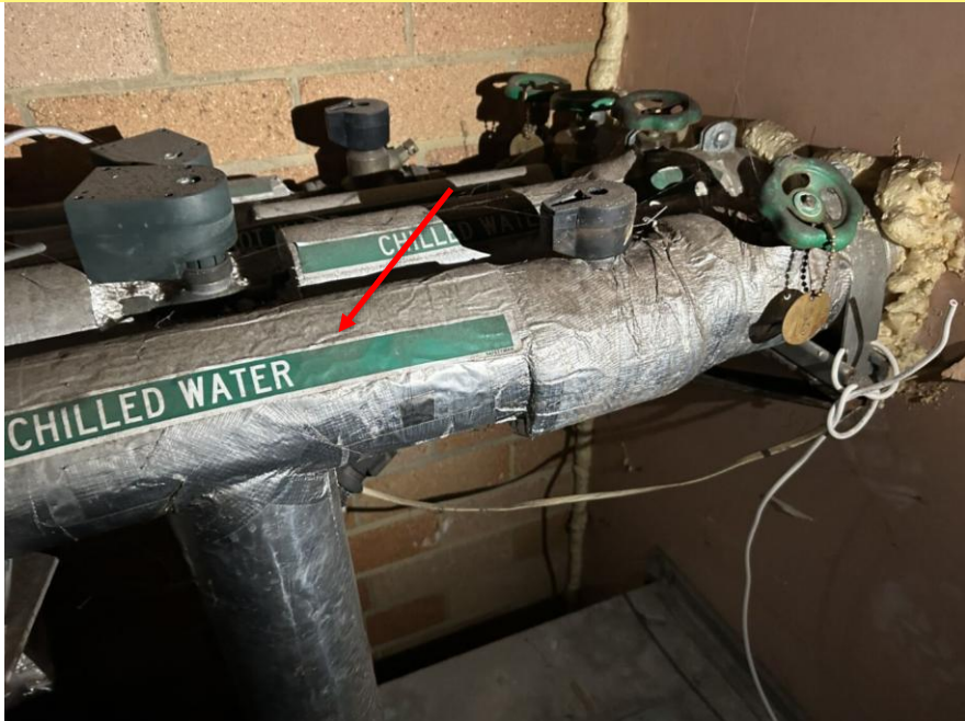
Photo 3: Assumed SMF insulation surrounding chilled water pipe in Centenary Hall
