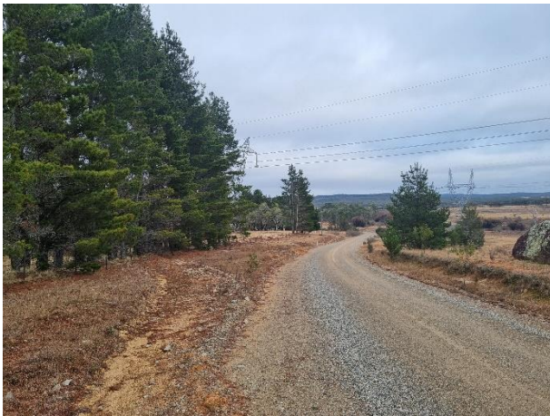
PHOTOGRAPH 5-9 DRAINAGE TRENCHES NORTH VIEW (ERM 2025)
