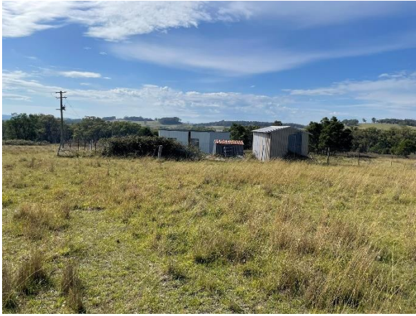
PHOTOGRAPH 5-5 SHEDS TO EAST OF DEVELOPMENT FOOTPRINT (ERM 2025)
