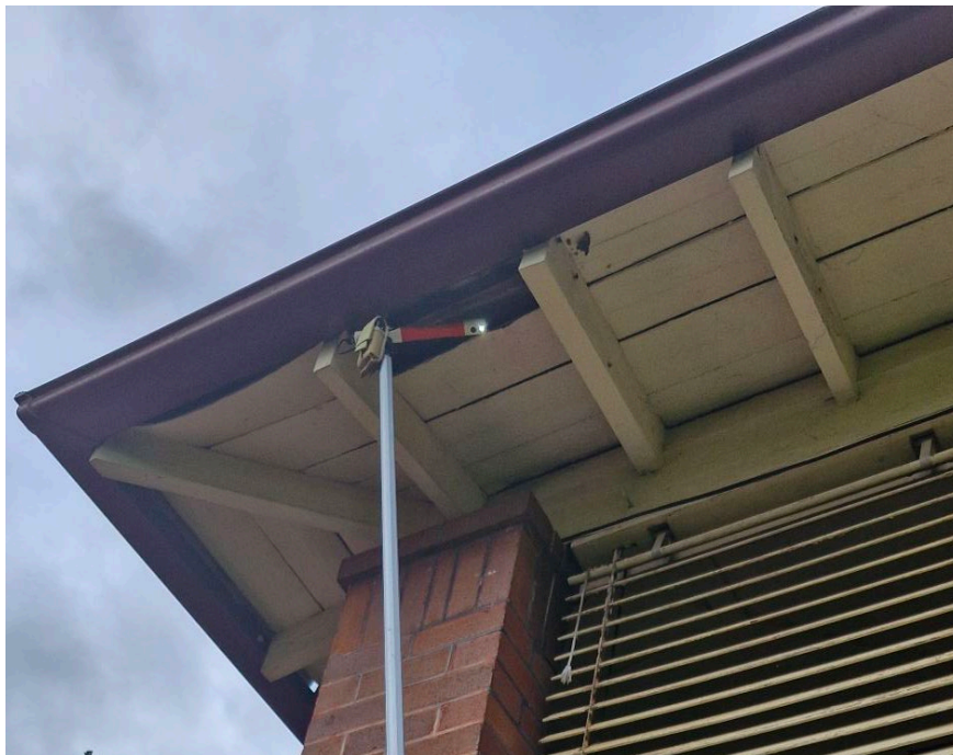
Photo 11 Inspection of the roof cavities were searched using a pole camera
