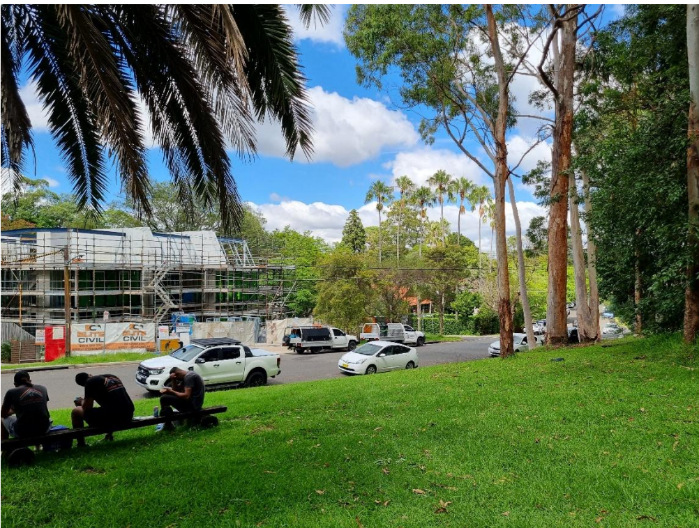
Figure 16 View of the terracotta tiled roof of the heritage item through trees from the park near Balfour Street looking southwest.
