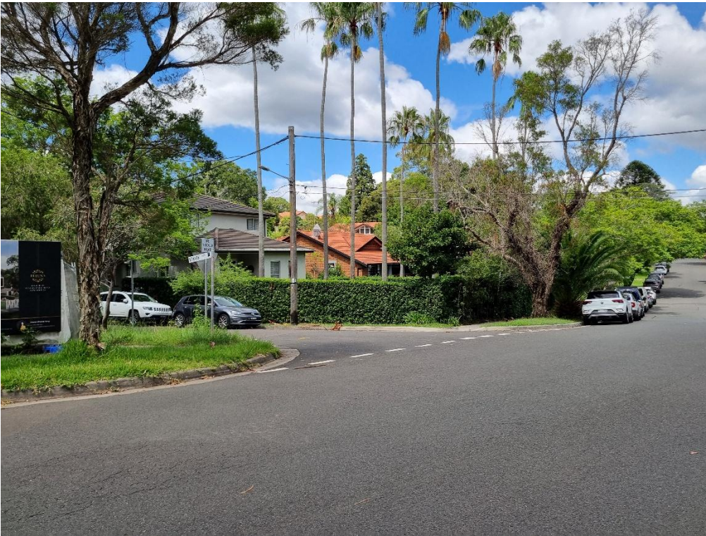
Figure 15 View of the heritage item, 28 Bent St from the park looking southwest
