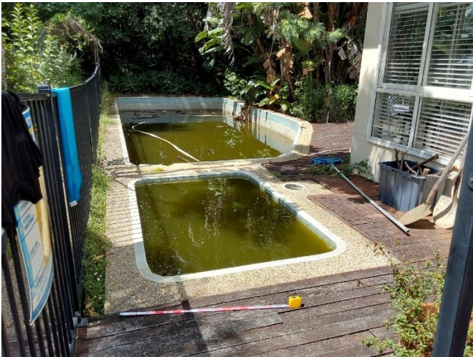
Photo 34 Facing south in 16 Bent Street showing the Newark swimming pool [9]
