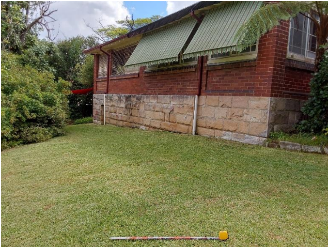
Photo 16 Facing northeast in 14 Bent Street showing the house [1]
