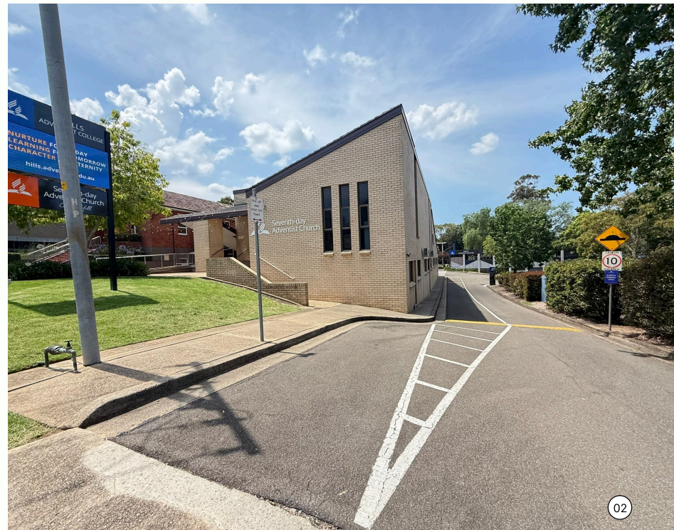
Cecil Ave - North Facing
