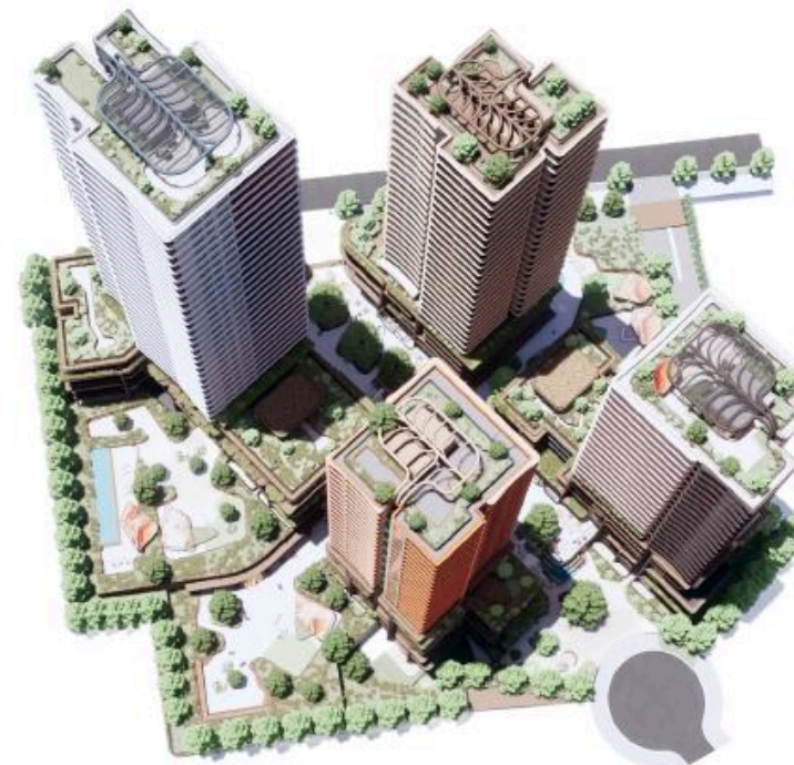
Figure 4: Aerial view from A+ Design Group
