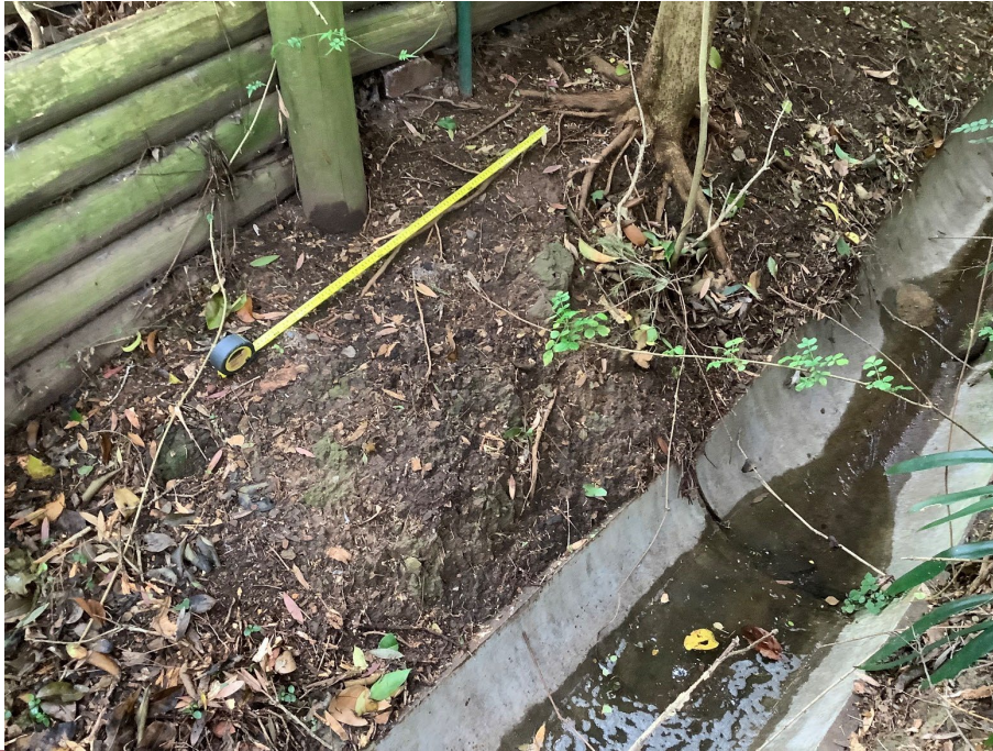
Figure 5-9: Stormwater overflow channel at Lot DP531559. Scale at one metre.
