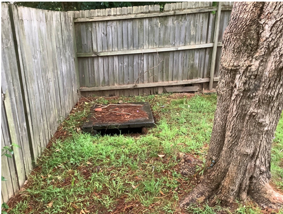
Figure 5-10: Stormwater drain at Lot DP15399.
