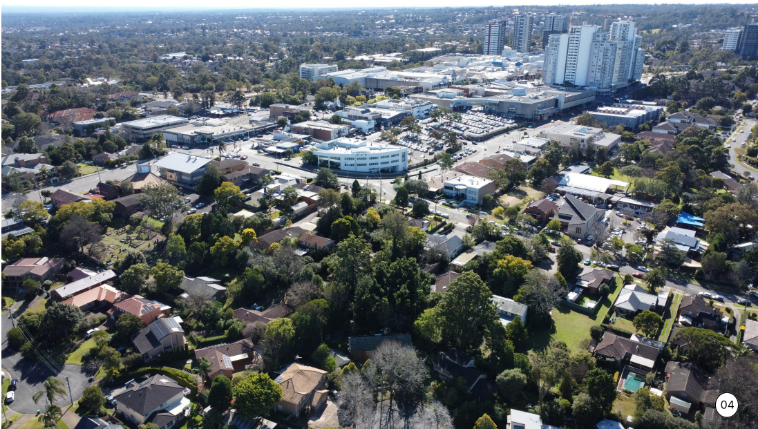
Roger Ave - Aerial North West Facing
