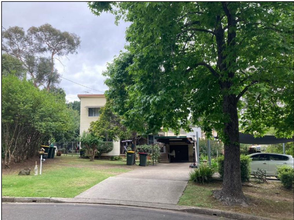
Figure 13: An example of a two-storey mid-to-late 20 th century period dwelling to the southeast of the site on Roger Avenue.
