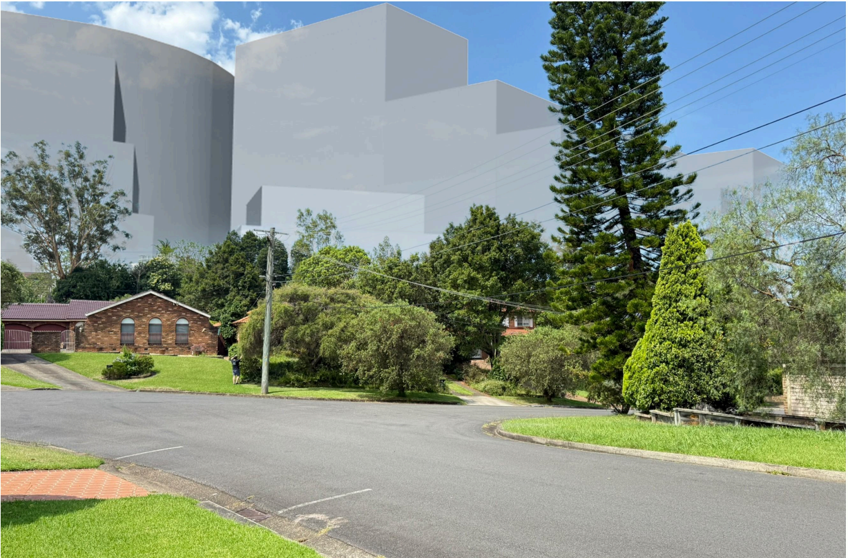
Photomontage of new proposal with 'future character' proposal in reference to The Hills Shire Castle Hill Precinct Plan in transparent grey
