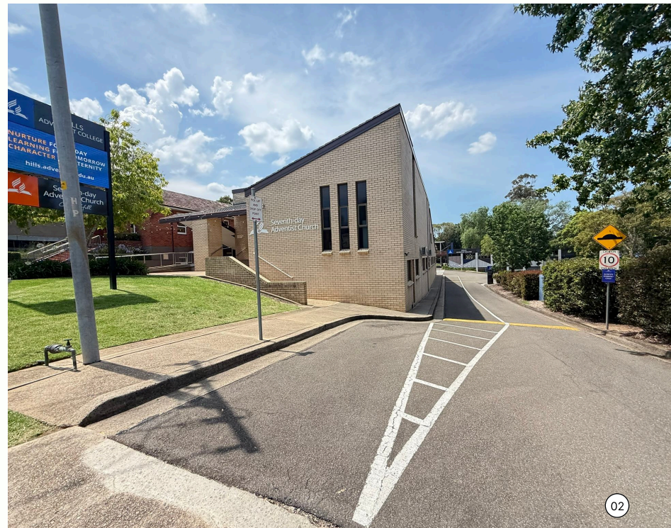
Cecil Ave - North Facing
