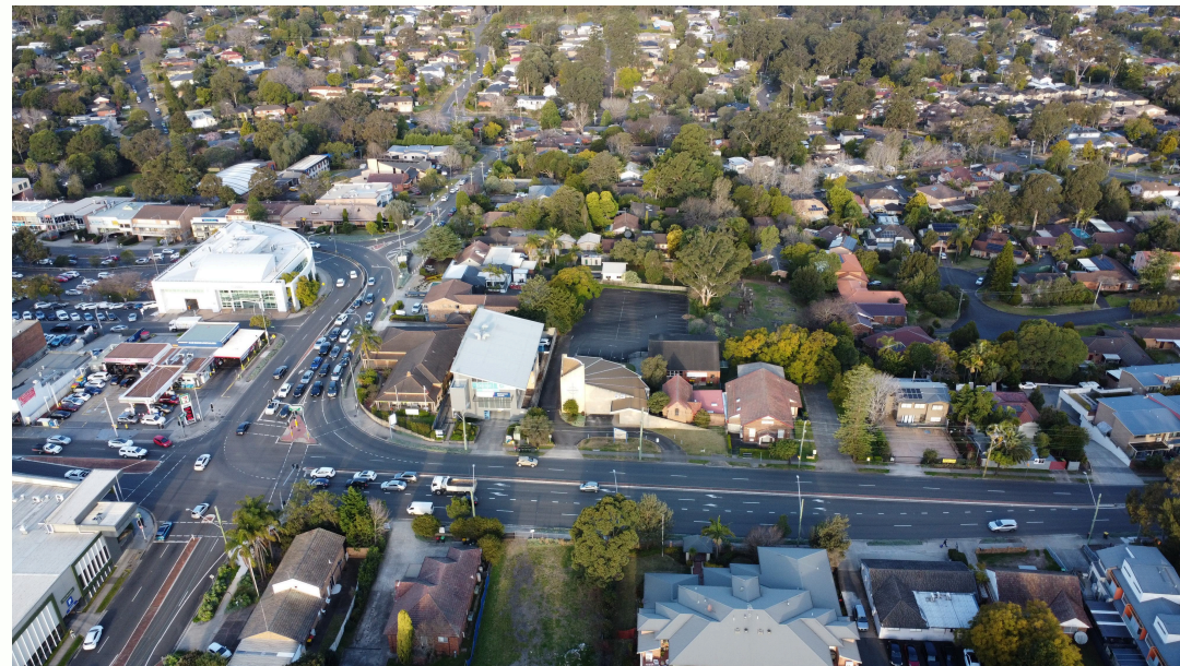
Old Northern Road - Aerial East Facing
