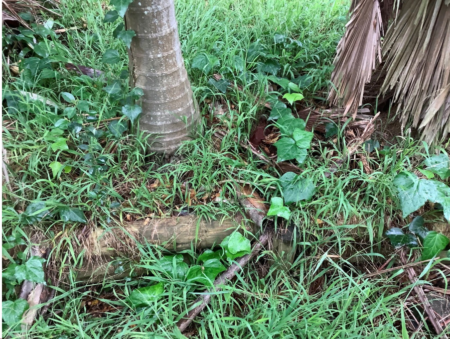
Figure 5-1: Retaining wall present in Lot DP547897. Note ground surface visibility is 0%. Height of the retaining wall is 40 mm.
