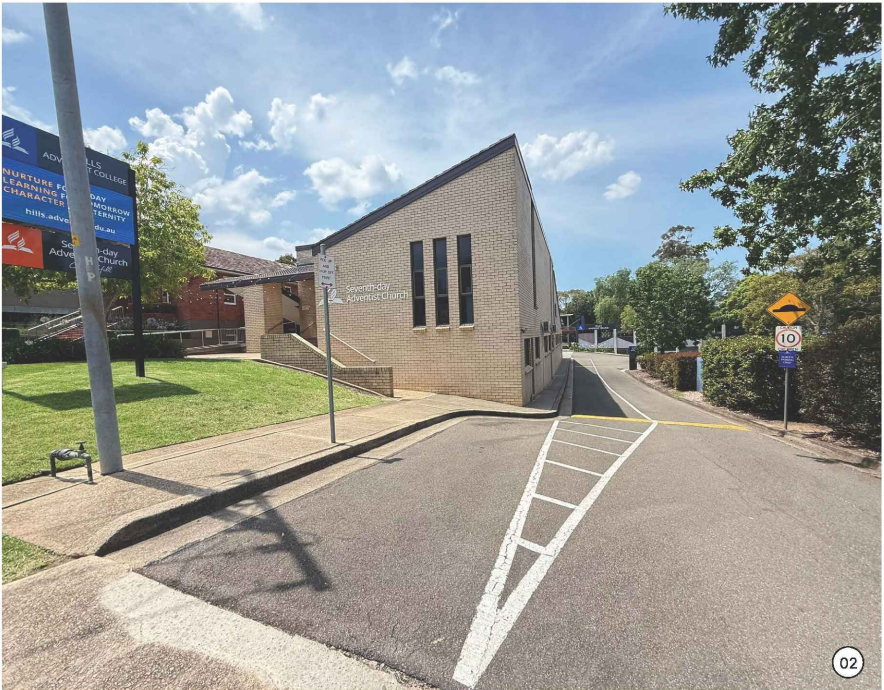
Cecil Ave - North Facing
