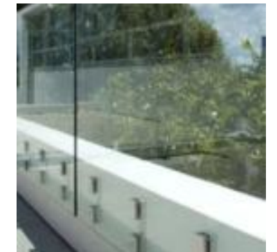
GLASS BALUSTRADE PIN FIXED TO UPSTAND
