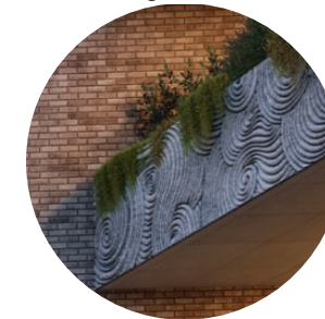
3. Balcony spandrel with Dharug Cultural motifs cast in concrete
