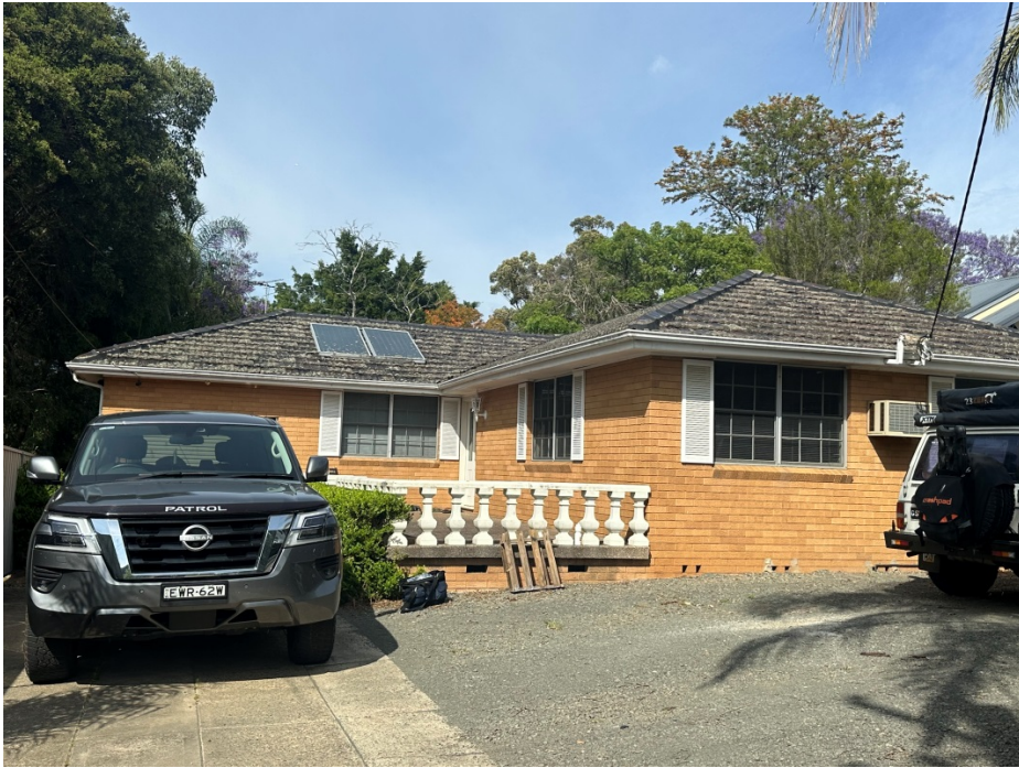
Photograph 25: 103 Cecil Avenue (Lot 1 in DP 547897; 810m 2 )
