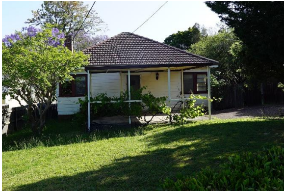
Figure 3.11 99 Cecil Avenue appears much older than the other pre-1943 buildings extant on the site. Later modifications may obscure older fabric. Facing south.
