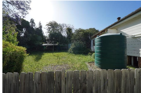
Figure 3.12 The rear of 99 Cecil Avenue shows minimal modification. Facing west.
