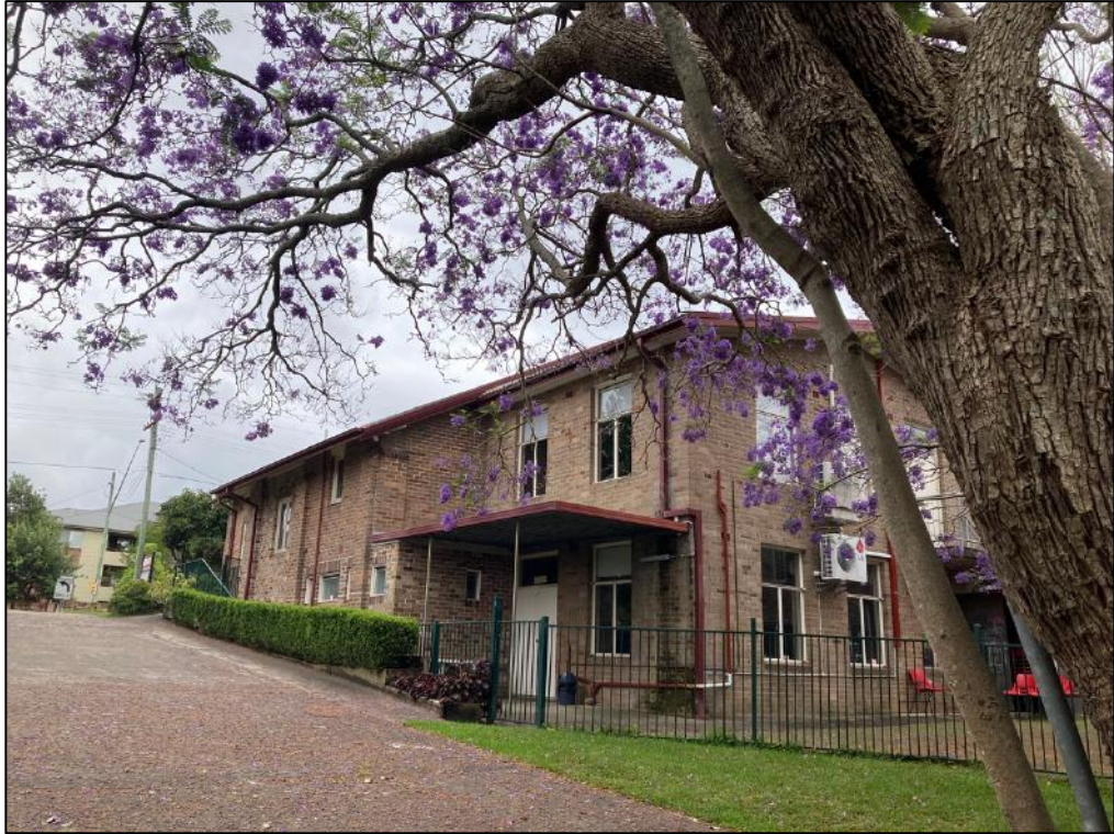
Figure 18: The southern and rear elevations of the 'Christadelphian Church', as viewed from the driveway.
