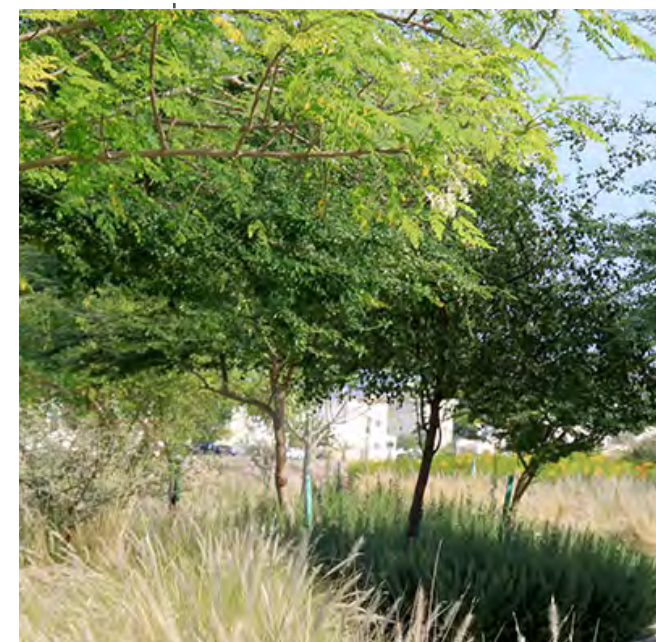
Vegetation on top of retaining wall
