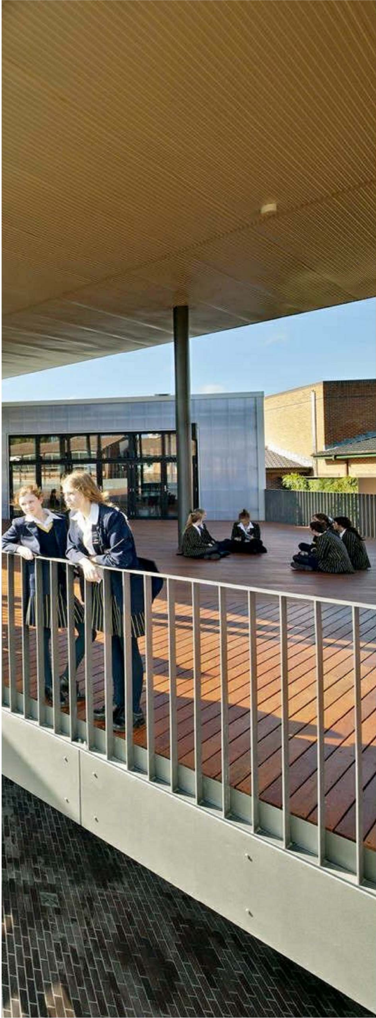
BAL - METAL SHEET WITH VERTICAL FLATS
