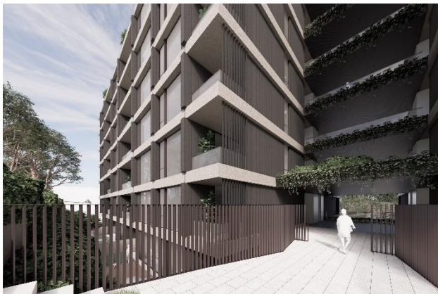
View of pedestrian entry and open lobbies.
