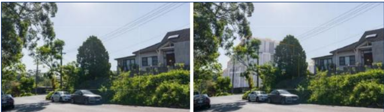
Figure 12 | Existing (left) and proposed (right) view from 4 Maclaurin Parade (Source: Amendment Report)
