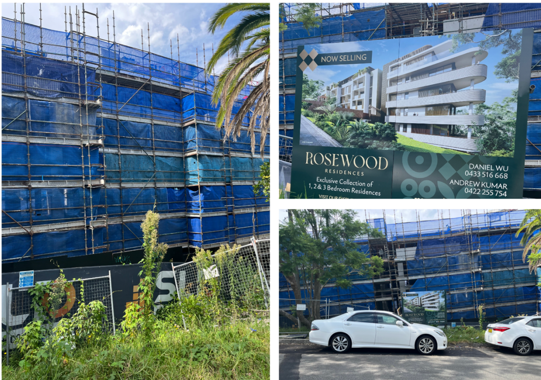
Figure 6 New apartment buildings being built in the immediate area (source: Forward-Thinking)
