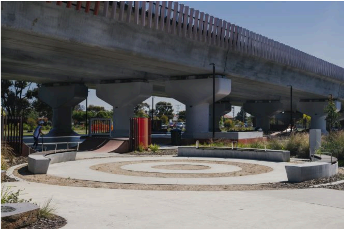
Level Crossing Removal Project, Melbourne: Integrated seating forming a Yarning Circle, Photography: Sarah Pannell.
