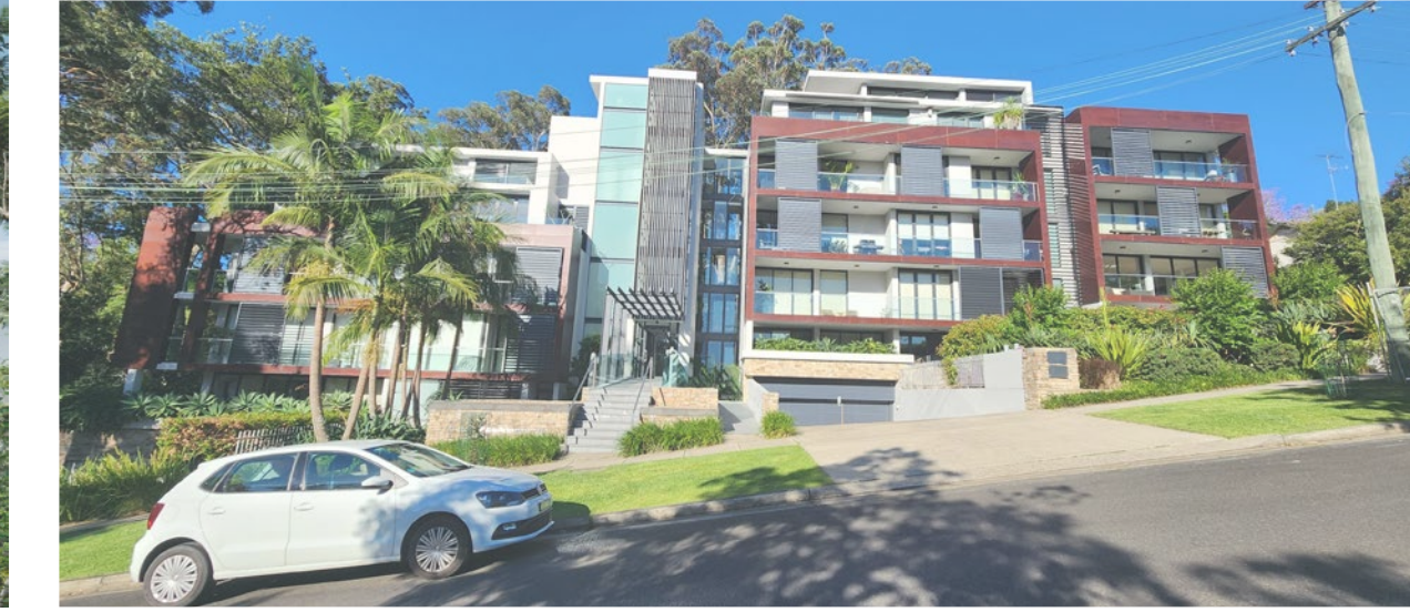
02 Kings Apartments, 9-15 Kings Avenue
