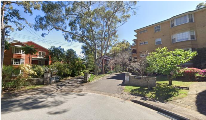
Figure 4 6 and 10 Larkin Street, Roseville (Google maps)
