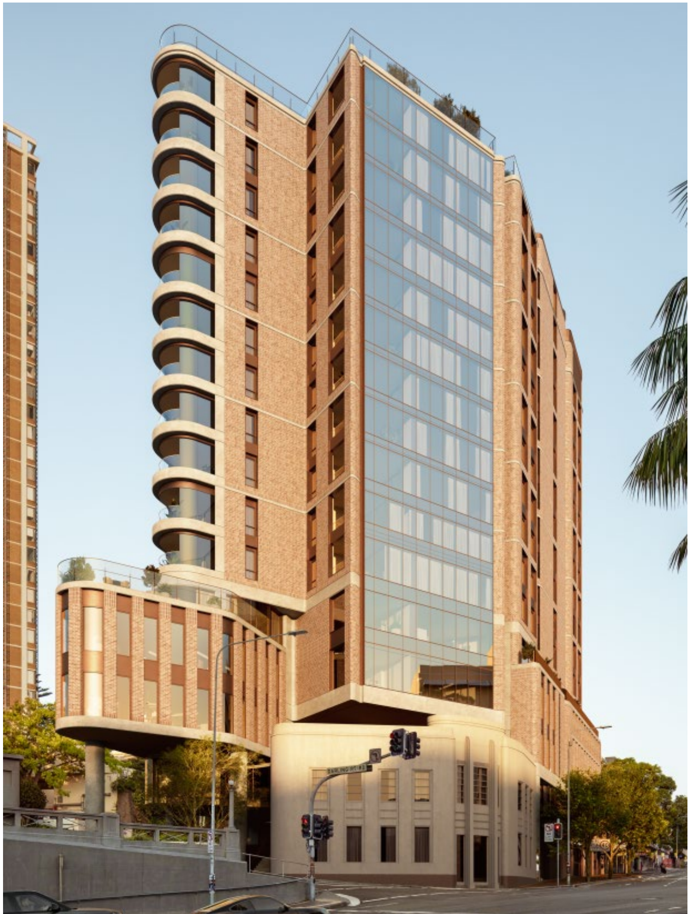
Figure 1 The development looking north-east along New South Head Road
