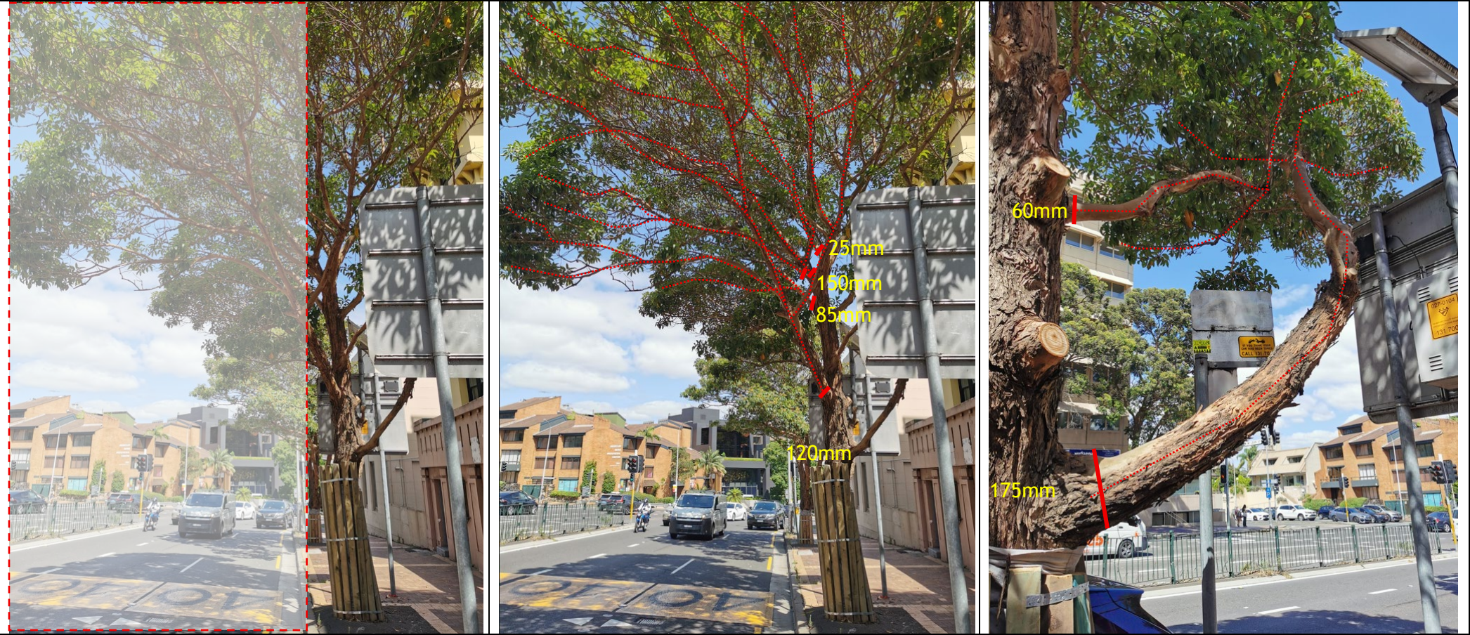
Figure 9- Tree pruning requirements for tree two (2).
