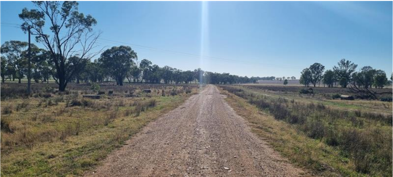
Figure 1-5 View from the existing access point off Holbrook Road facing east along the site access road
