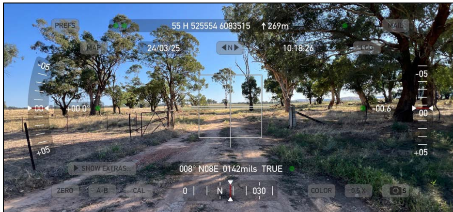
Photo Point R. Showing the general condition of the existing/proposed internal property access road route heading towards the Mangoplah BESS Project Site. (Hague, 2025)
