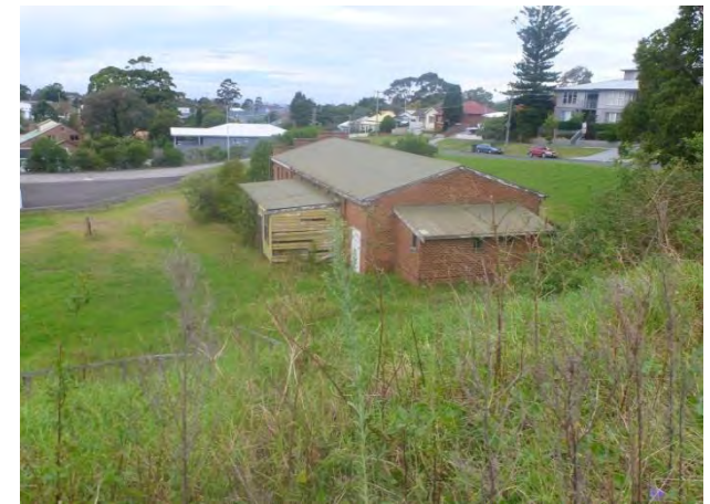
Figure 6: View east from western lot (Part Lot 1 DP 165903) to building proposed for demolition
