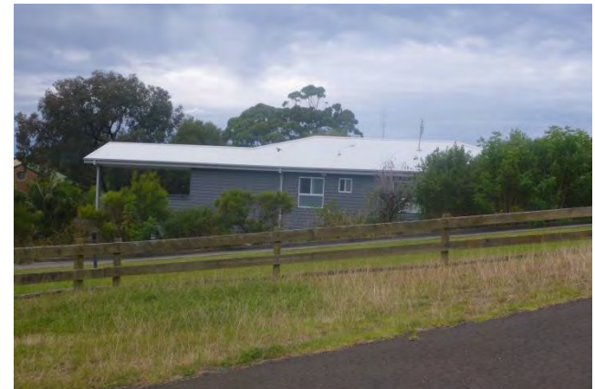
Figure 15: View of dwelling house directly adjoining the site to the east on Hospital Road
