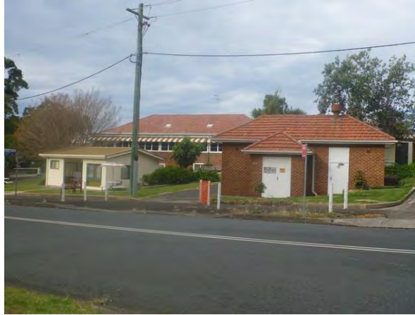
Figure 11: Additional view of Bulli Hospital located on the southern side of Hospital Road directly opposite the subject site
