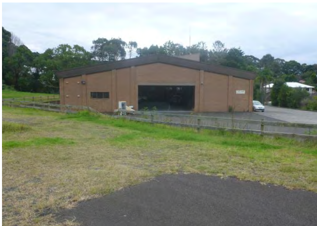
Figure 7: Existing ambulance station proposed for future excision from Lot 1 DP 175787
