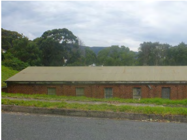
Figure 5: View north from Hospital Road to subject site and building proposed for demolition on Lot 1 DP 175787
