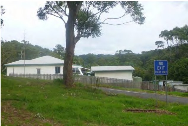
Figure 13: Development in the vicinity of the subject site directly to the west on Hospital Road
