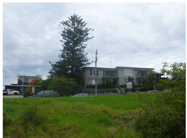
Figure 12: Development in the vicinity of the subject site opposite to the south on Hospital Road (Source: TCG Planning, June 2016)
