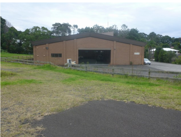
Figure 11: Existing ambulance station proposed for future excision from Lot 1 DP 175787 (Source: TCG Planning, June 2016)
