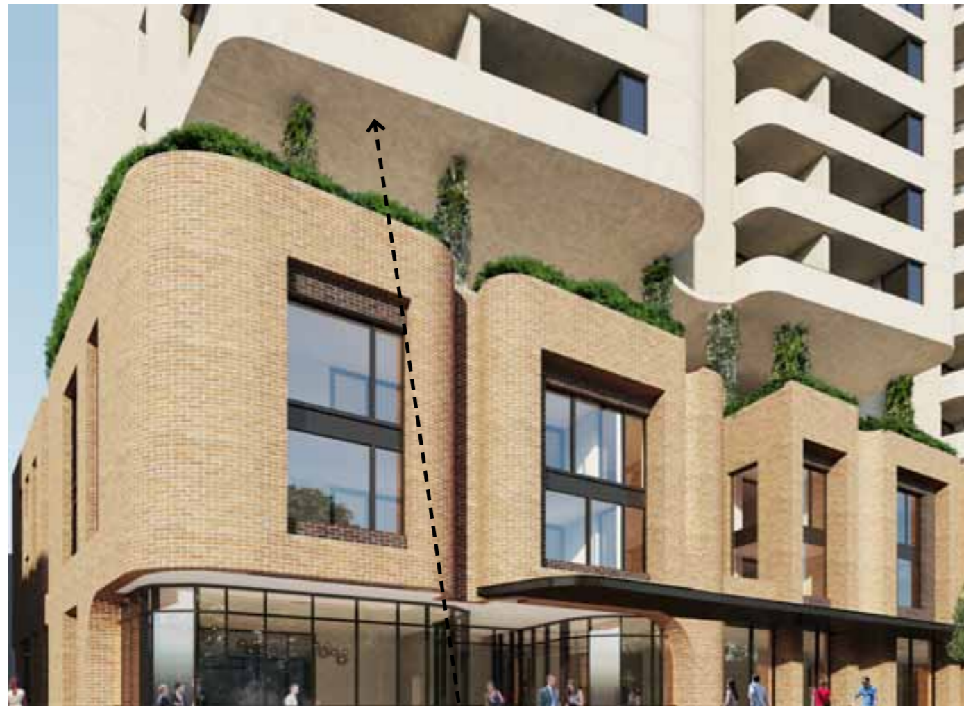
Location 1 Designed panels fixed to the soffit of Level 3 communal open space.
