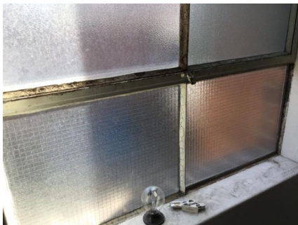
PHOTO NO.: J155653-001-PHOTO028 RESULT: LEAD (PAINT) - POSITIVE, 1.1% W/W BUILDING/LEVEL: MOWERS SHED - LEVEL ONE ROOM/LOCATION: ALL AREAS - WINDOW FRAMES FEATURE/MATERIAL: WINDOW FRAME - UPPER & LOWER PAINT SYSTEM/S SAMPLE NO.: J155653-001-LP-006
