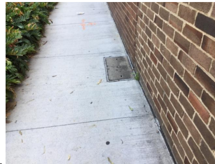
PHOTO NO.: J155653-001-PHOTO024 RESULT: ASBESTOS - PRESUMED POSITIVE BUILDING/LEVEL: MAIN BUILDING - GROUND LEVEL ROOM/LOCATION: PAVEMENT - ADJACENT OUTSIDE WALL FEATURE/MATERIAL: TELECOMMUNICATIONS PIT - MOULDED FIBRE CEMENT SAMPLE NO.: NOT SAMPLED RESTRICTED ACCESS
