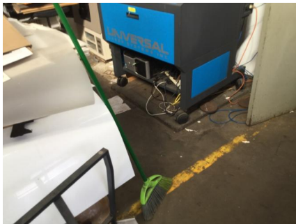
PHOTO NO.: J155653-001-PHOTO027 RESULT: STORAGE TANKS - PRESUMED POSITIVE BUILDING/LEVEL: MOWERS SHED - GROUND LEVEL ROOM/LOCATION: MAIN SHED - BELOW FLOOR FEATURE/MATERIAL: NON-HAZARDOUS FEATURE - NON-HAZARDOUS MATERIAL SAMPLE NO.: NOT SAMPLED NO ACCESS TO AREA BELOW FLOOR
