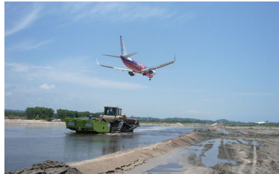
Figure 17. Construction earthworks can create temporary, but significant, wildlife attractants.
