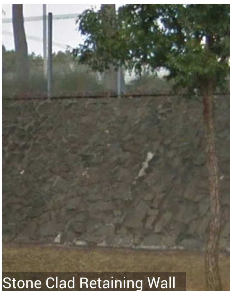
Stone Clad Retaining Wall
