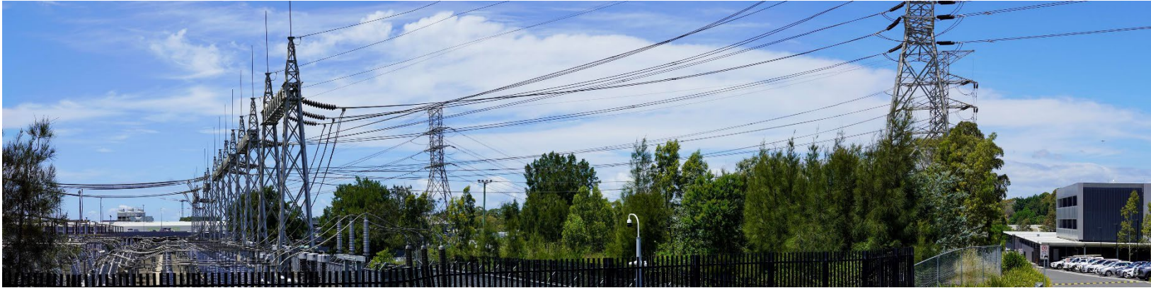
Figure 6.5-3: VP1 – M4 Western Motorway on-ramp (Aurecon, 2025)
